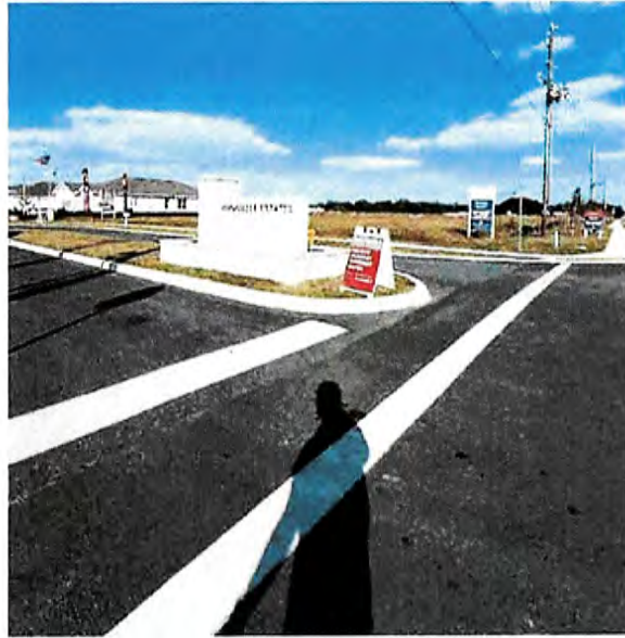
View of entrance to Annabelle Estates from Old Bartow-Lake Wales Road
